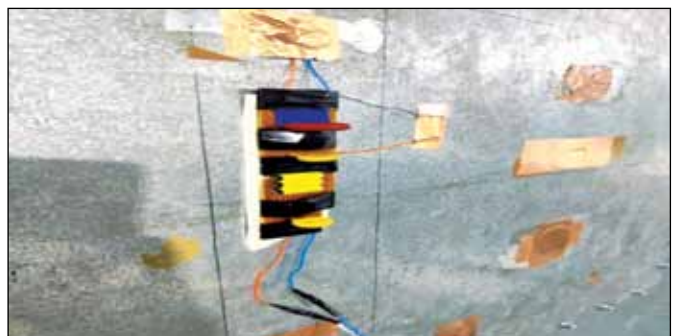
Single-phase Power Line Point-of-Entry (POE) protection HEMP filter
