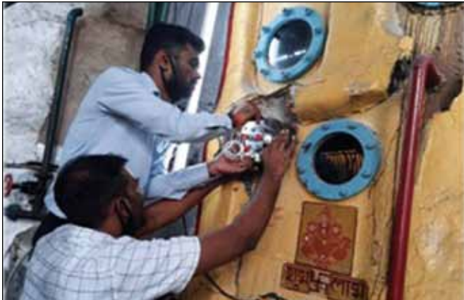
BRIX sensor installation at site
