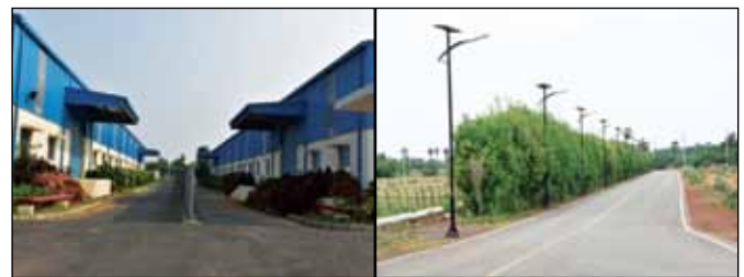
RBF Road Network and Landscaping Site Pics: EMC Sri City (Andhra Pradesh)
