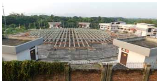
ST Radar site
