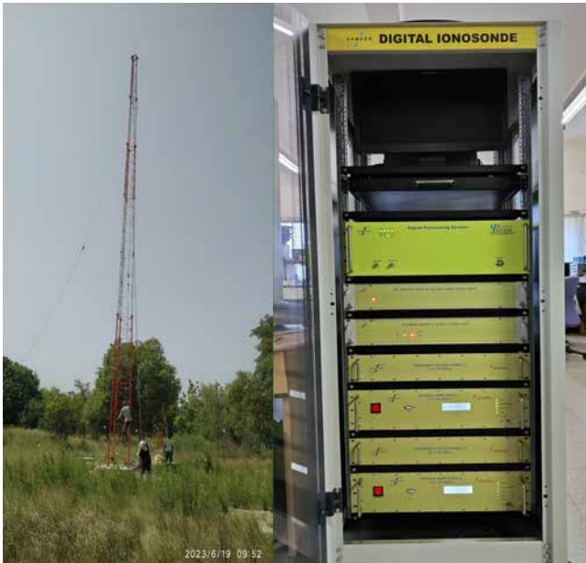
Fig: Transmit antenna tower and ionosonde control room hardware
